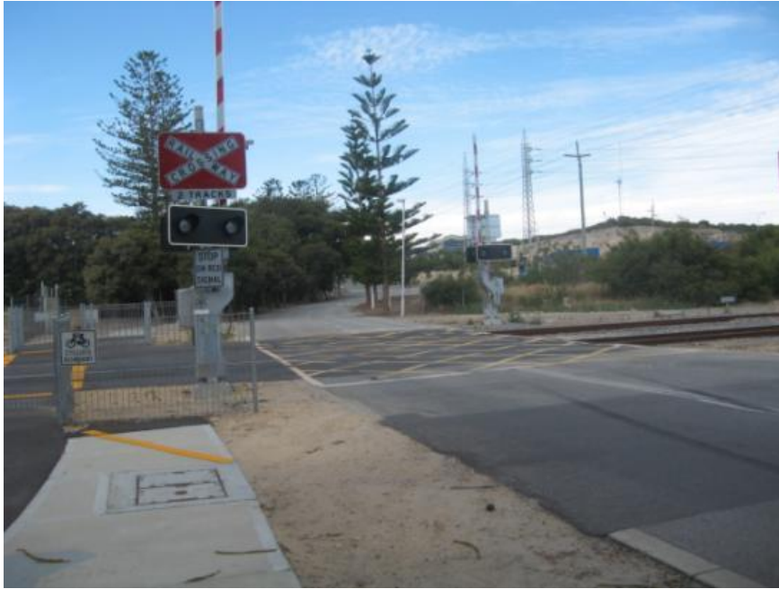
Photo 3.1 McTaggart Cove rail crossing
