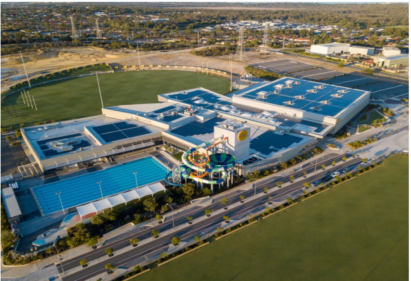
Image 2: Solar photovoltaic system (1MW) on the Cockburn ARC
