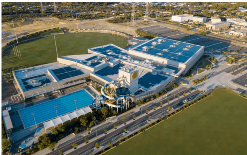
Image 1: Solar photovoltaic system (1MW) on the Cockburn ARC
