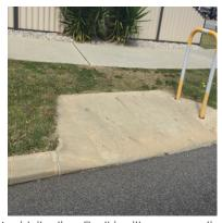
Avoid situations like this with no connection between dropped kerb ramp and footpath
