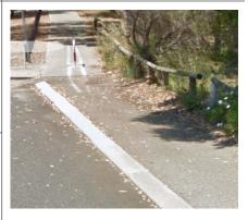
Kerbed, unmarked two-way cycle path, Windelya Road, Kardinya
