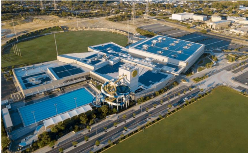
Image 1: Solar photovoltaic system (1MW) on the Cockburn ARC
