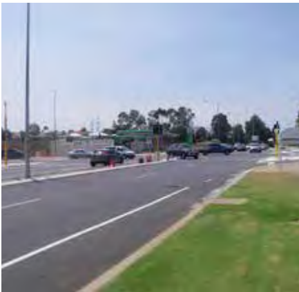
Above: Ongoing road upgrades
