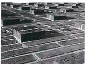
relief brickwork
