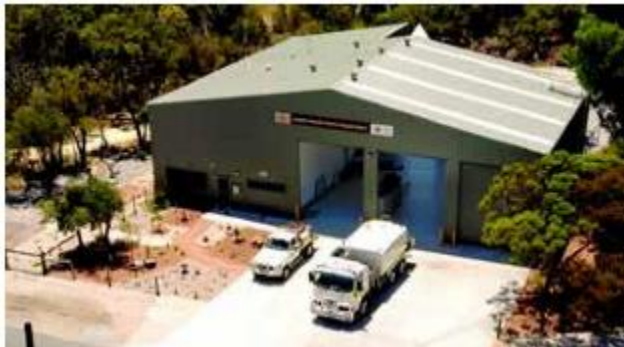
Jandakot Volunteer Bush Fire Brigade station - January 2020
