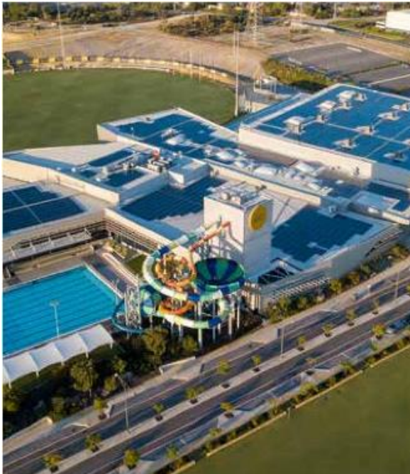
Solar panels installed at Cockburn ARC
