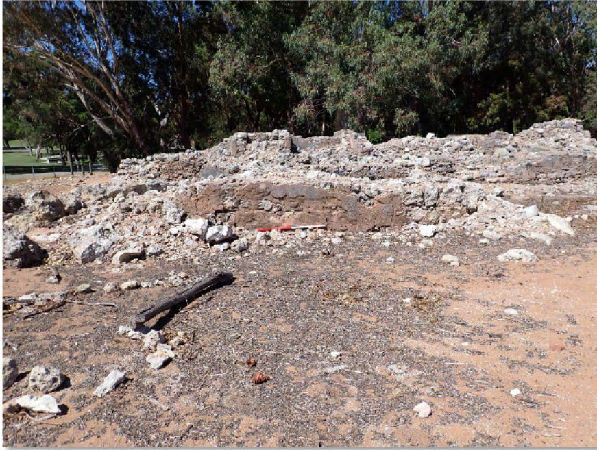
Figure 34. Western wall of the Davilak house building within the Davilak Ruins Complex – Eastern Section
