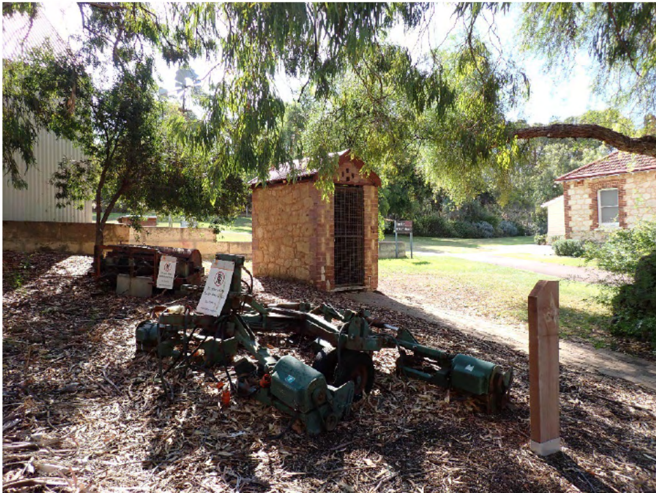
Figure 53. Stone water closet
