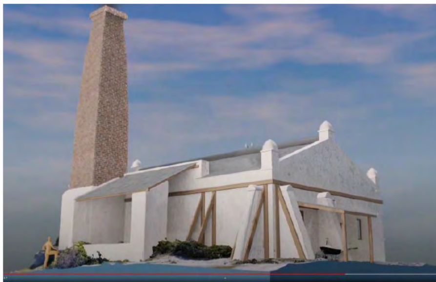
Figure 46. 3D reconstruction of former salt works on Rottnest Island. Circa. 1898 based on 3D photogrammetry, historic plans, and contemporary photographs.
