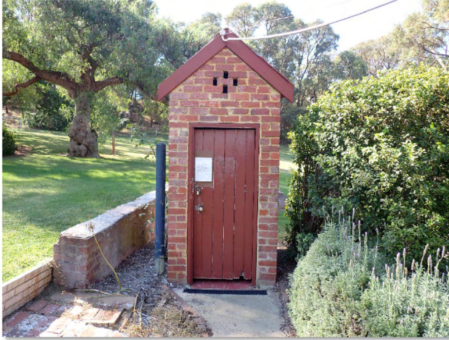
Figure 54. Brick water closet
