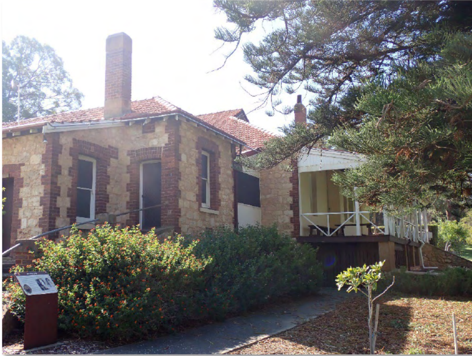
Figure 50. View northwest of the kitchen block and the wrap-around verandah
