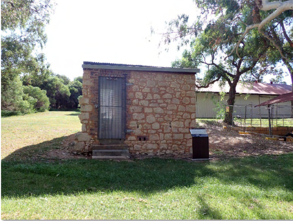
Figure 52. Single-roomed stone building
