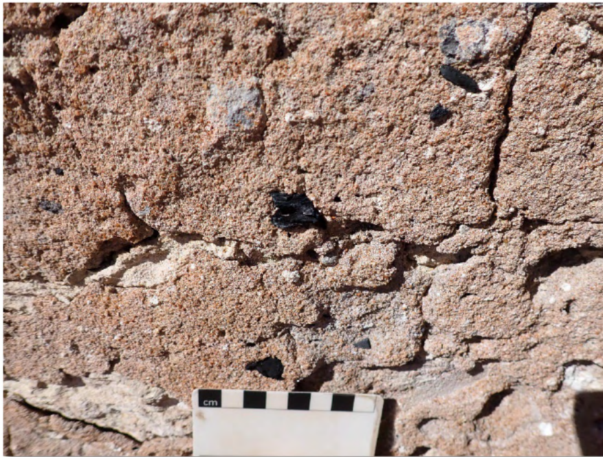
Figure 39. Piece of charcoal embedded in the mortar of a wall in the Davilak Ruins Complex – Northwestern Section
