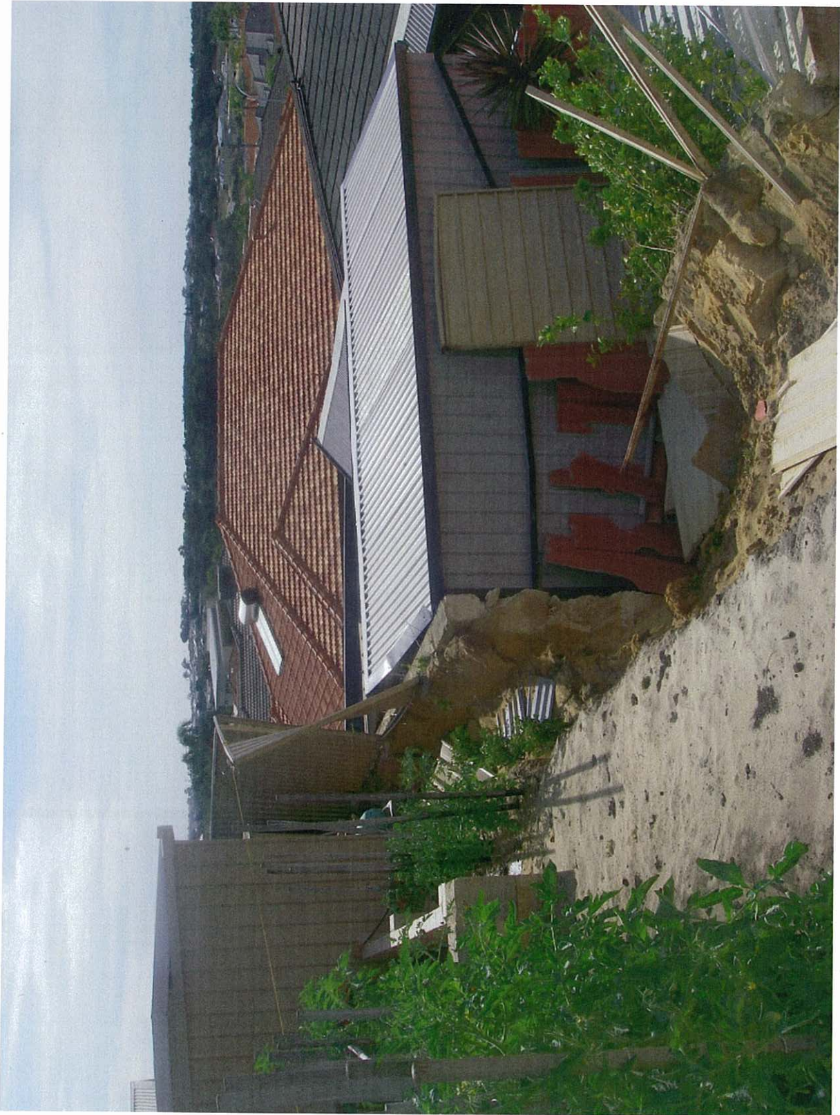
View of collapsed section of partially collapsed wall from No. 46 Fairbairn looking down into No. 14 Carrello.
