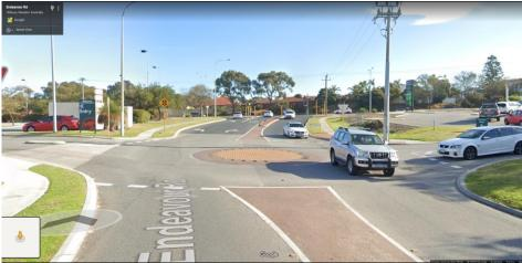
Picture 2 - Mini Roundabout with fully mountable inner circle – Endeavour Road, looking north towards Whitfords Avenue, City of Joondalup
