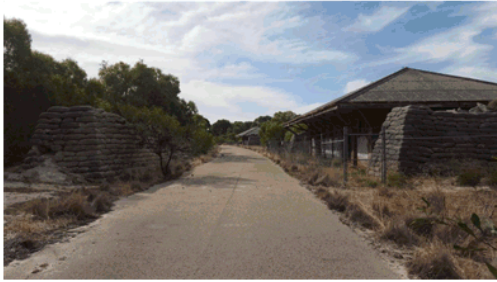
Figure 27. Remaining munition magazines, Woodman Point
