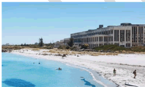
Figure 30. South Fremantle Power Station
