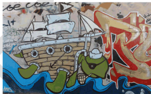
Figure 31. Graffiti within the interior of the South Fremantle Power Station
