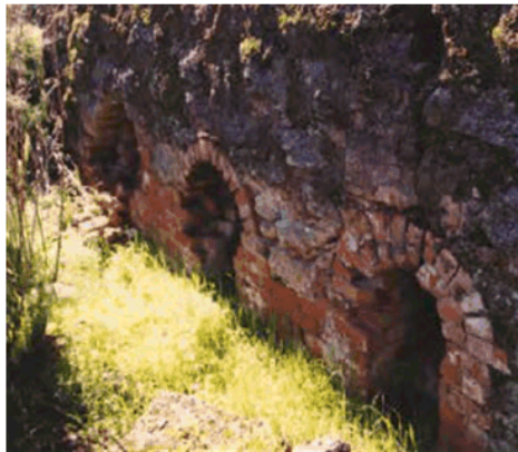
Figure 46. Lime Kilns, Munster
