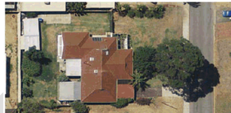
Figure 9. Infill development (Spearwood) demonstrating reduced landscaping and increased hardstanding with redevelopment (top photo)
