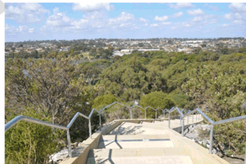
Figure 59. Manning Park stairs
