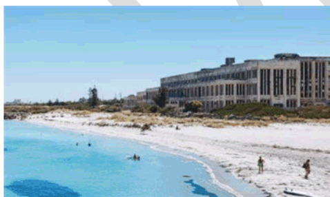
Figure 30. South Fremantle Power Station
