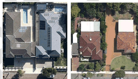
Figure 10. Example of replacement single dwellings in Perth Metropolitan area demonstrating greater site coverage and loss of landscaping without infill or higher residential codings
