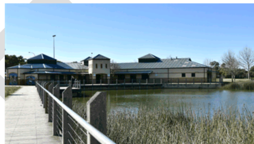
Figure 36. Beeliar Community Centre
