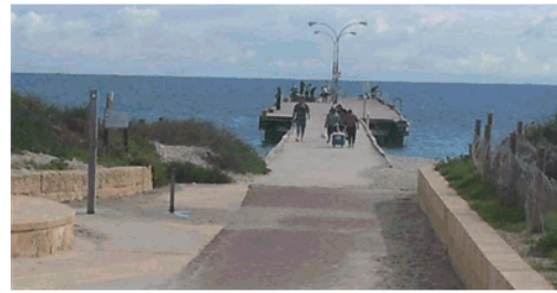
Figure 29. Magazine Jetty, Woodman Point
