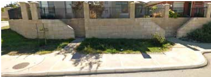
Figure 7. Disconnected verge before and after.
