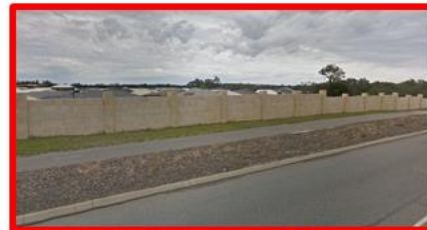
Existing noise wall to be extended
