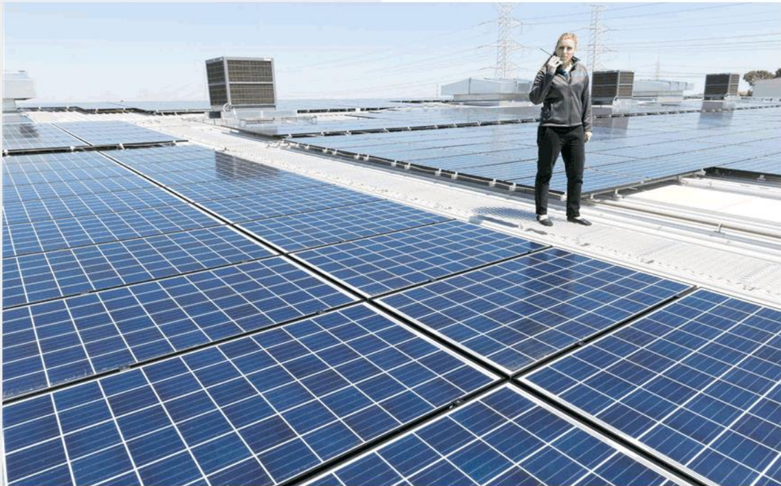
Above: Solar PV panels provide half the electricity for Cockburn ARC
