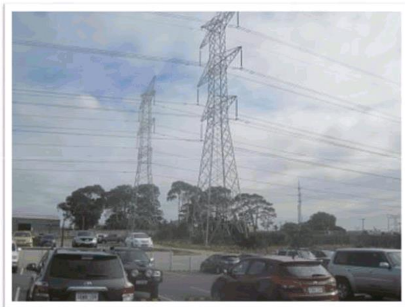
Adjoining Power Lines
