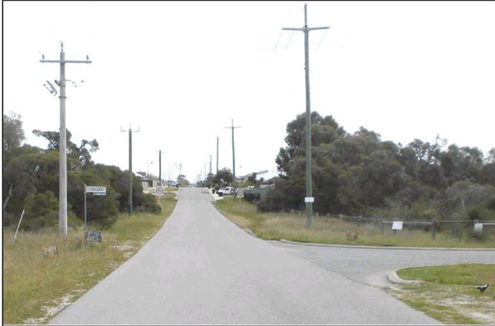
Note the 50km/h speed limit signs facing westbound traffic
