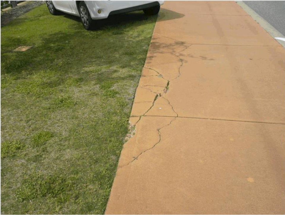
Photo 4: Looking east along Gaebler Road from Lyon Road
