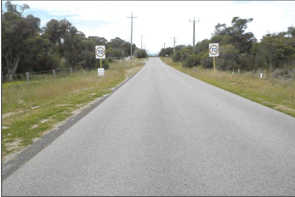
Photo 8: Looking west along Gaebler Road from near Hausen Ct
