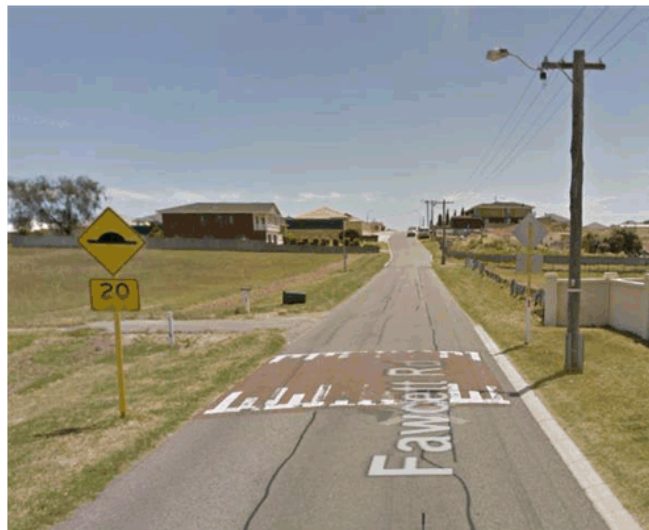
Figure 2 – Existing Speed Hump
