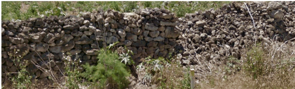
Figure 14. Intact section to the left, and collapsed section to the right
