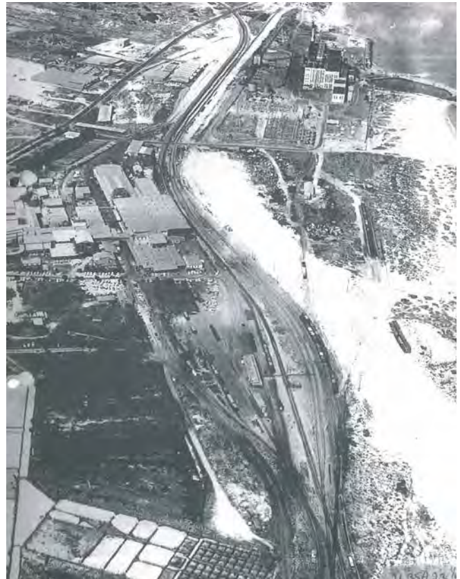
FIGURE 24 - AERIAL VIEW OF ROBB FREIGHT TERMINAL WITH SOUTH FREMANTLE POWER STATION IN BACKGROUND (UNDATED) SOURCE: MAUNSELL COLLECTION STATE LIBRARY OF WESTERN AUSTRALIA
