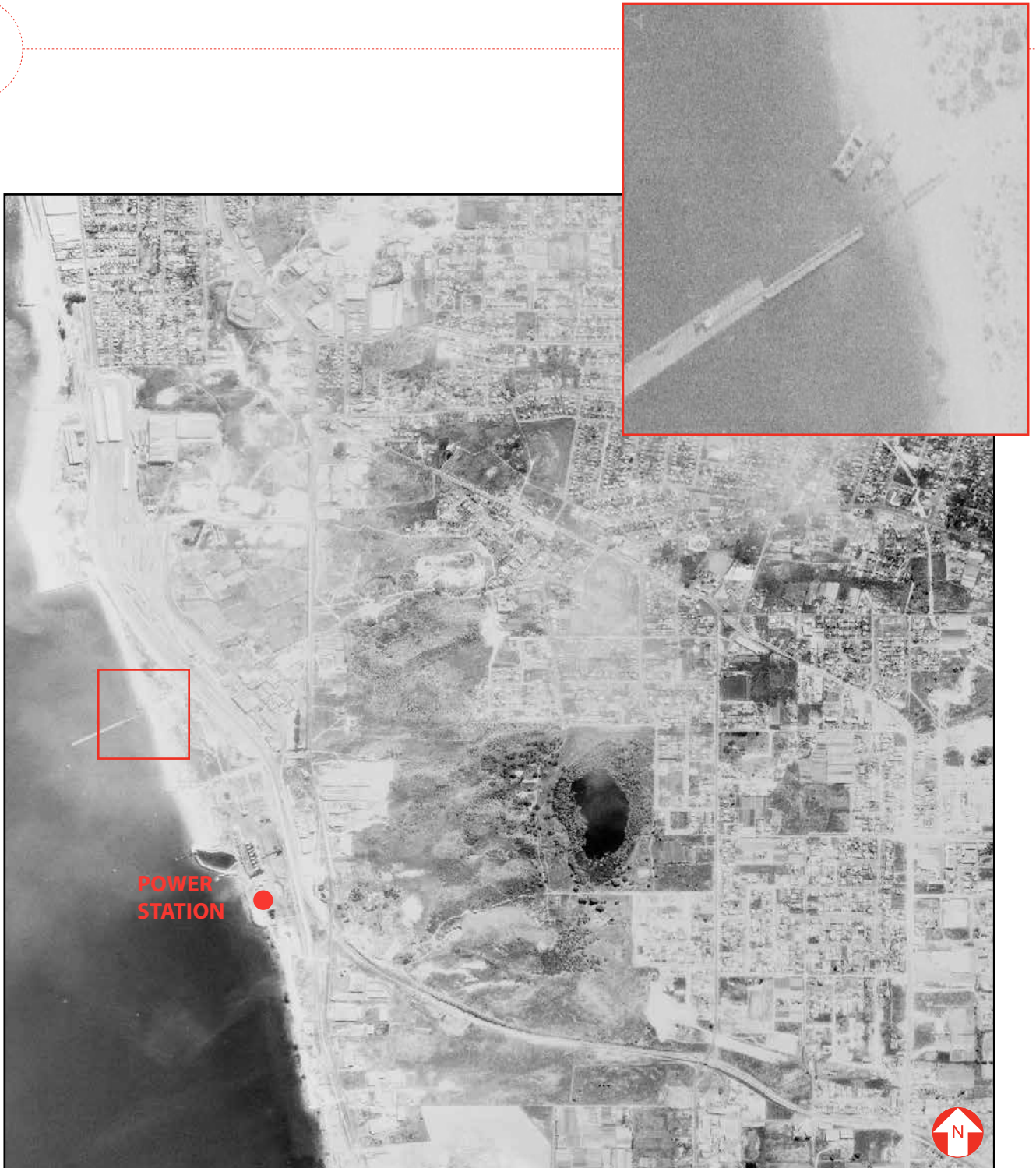
FIGURE 16 - AERIAL 1974 - INSET SHOWING WYOLA AND BARGE (REMAINS) ADJACENT TO ROBB JETTY, WHICH RAN ASHORE IN 1970
