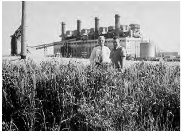
FIGURE 30 - SOUTH FREMANTLE POWER STATION (c1964) SOURCE: FREMANTLE CITY LIBRARY LOCAL HISTORY COLLECTION IMAGE NUMEBR 2497
