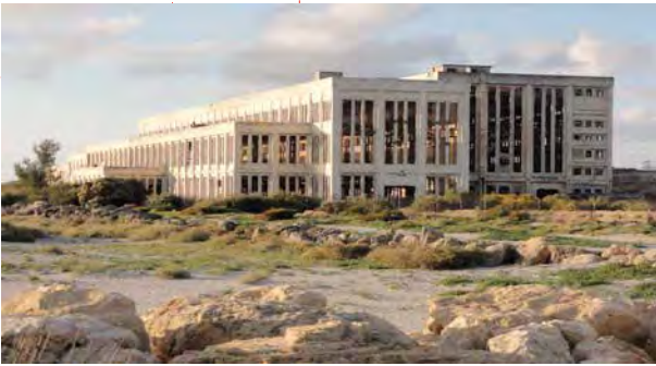
FIGURE 45 - SOUTH FREMANTLE POWER STATION
