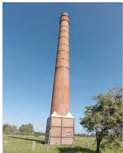
FIGURE 72 - ROBB JETTY CHIMNEY
