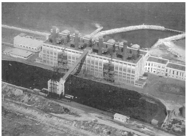
FIGURE 32 - SOUTH FREMANTLE POWER STATION (1955) SOURCE: EDMONDS, L; CATHEDRALS OF POWER PG 39
