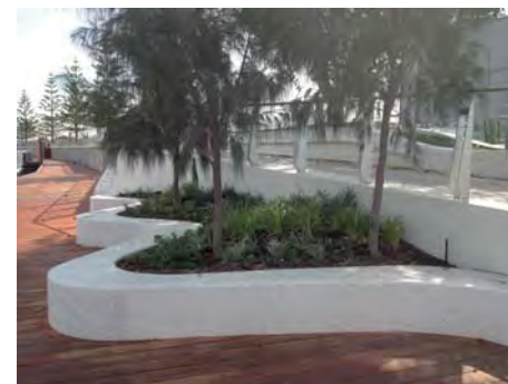
High quality finishes and detailing
