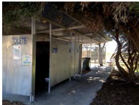
Toilet facilities at McTaggart Cove
