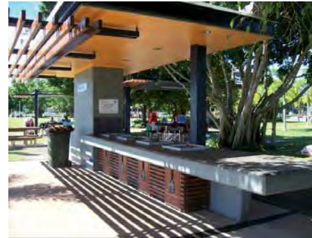
BBQ facilities integrated into custom designed shelter
