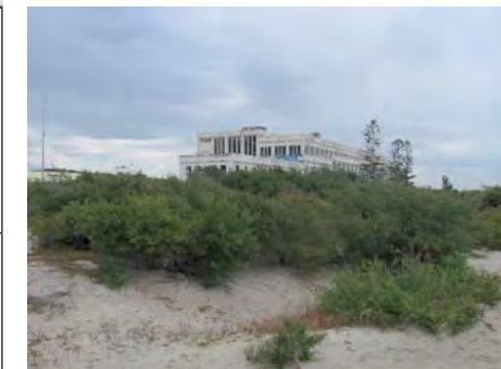
Invasive Tea Tree species in front of the Power Station
