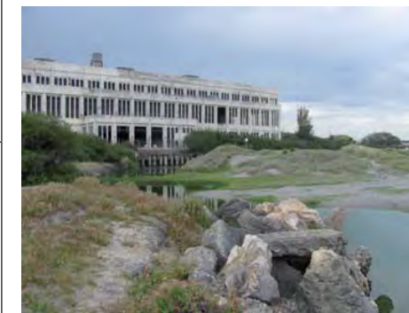
Mercury Contamination in front of the Power Station
