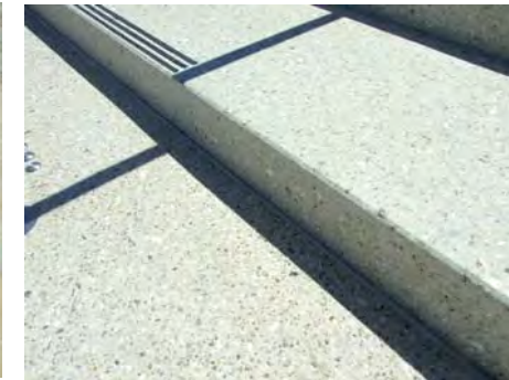
In-situ Exposed Aggregate Concrete
