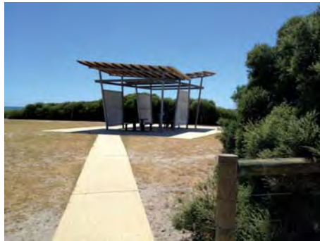
Existing shade shelters at Catherine Point
