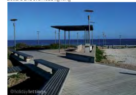
Boardwalk with integrated furniture, shelters and lighting
