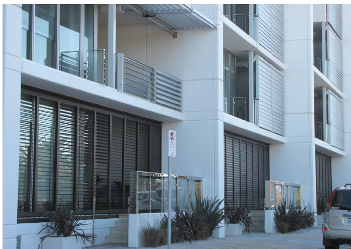
Well positioned balconies and windows to maximise surveillance
