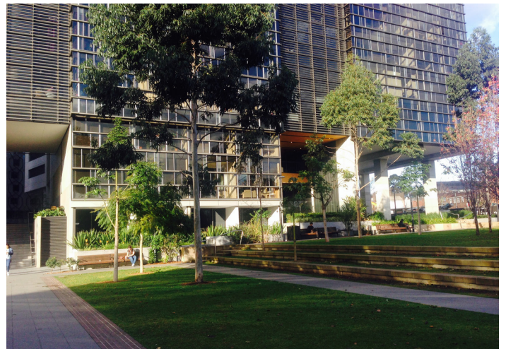
Planting at the building's ground level enhances the interface with the public realm
