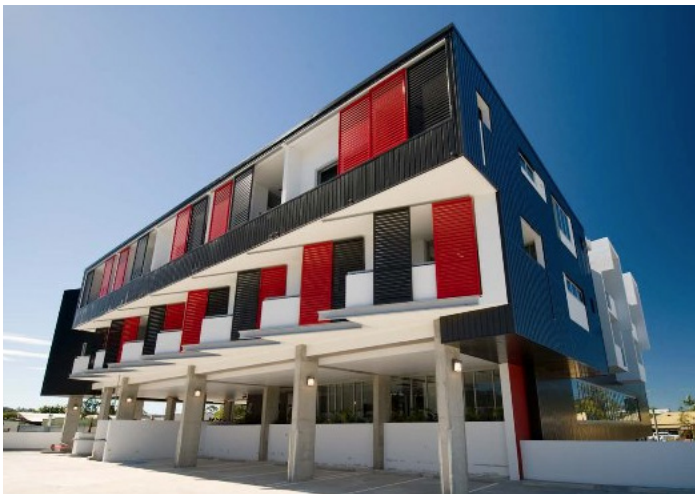
Undercroft parking to the rear of a site not visible from the street.
