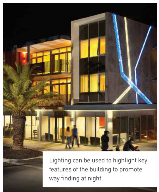
Lighting under overhangs and awnings promotes the feeling of safety at night.
