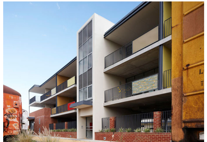
Example of a clearly defined pedestrian entry
