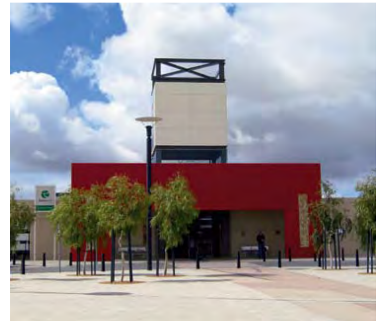
Cockburn Central Railway Station
