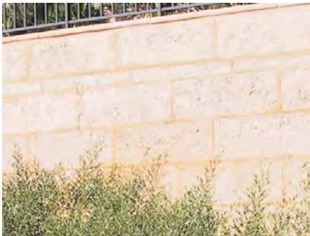
Limestone Retaining Wall
