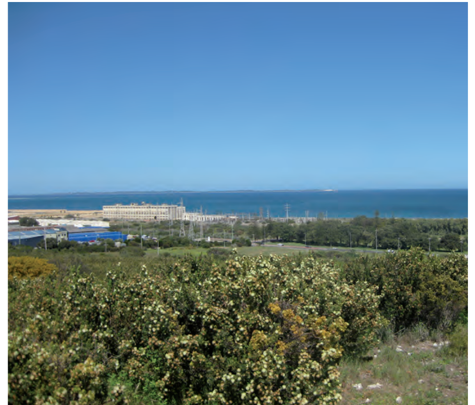
Bushland in Beelie Regional Park looking down at the Power Station
