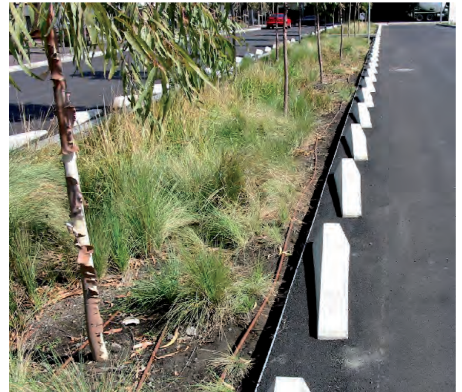
Planted swale median
