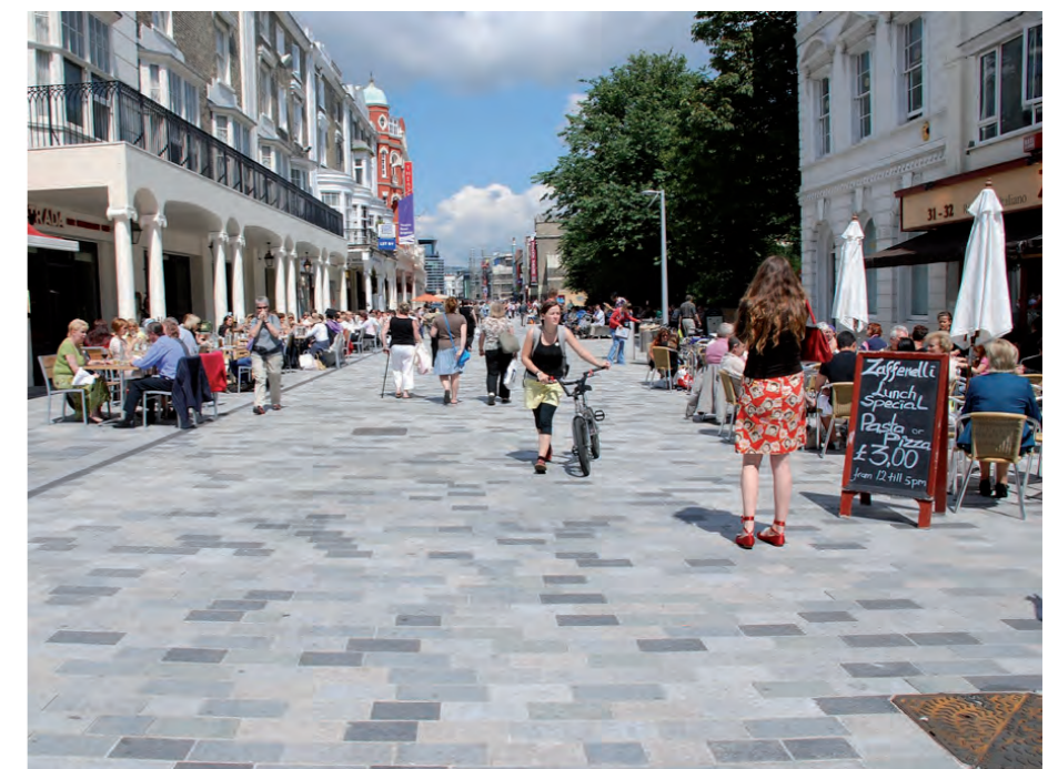
Example of a shared surface street where vehicles and pedestrians share the street
