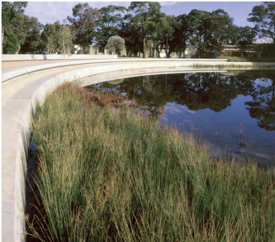
An example of a detention basin
