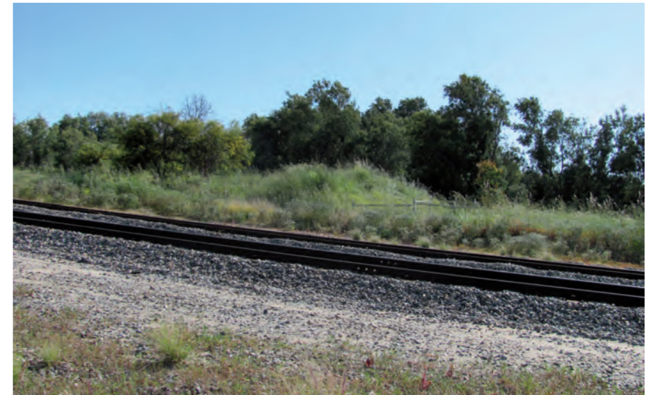
Freight rail infrastructure running through the site
