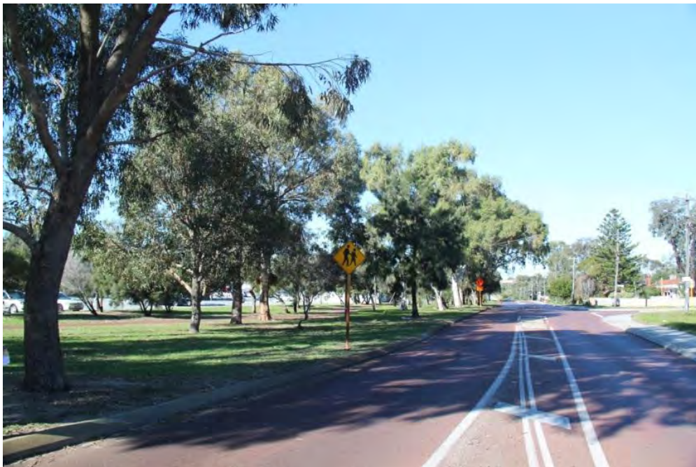
Image: Coolbellup Drive looking South.
