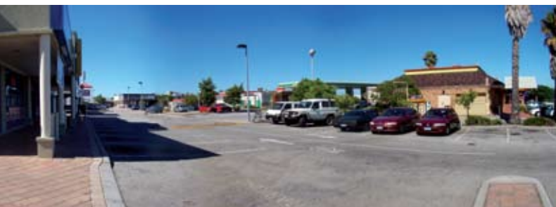
BEFORE – Car park dominated vista with little or no amenity or visual attractiveness.
