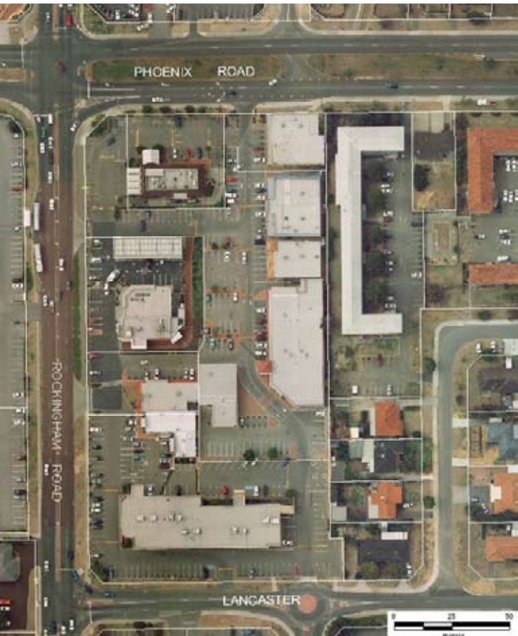
Aerial photo of the northern commercial end
