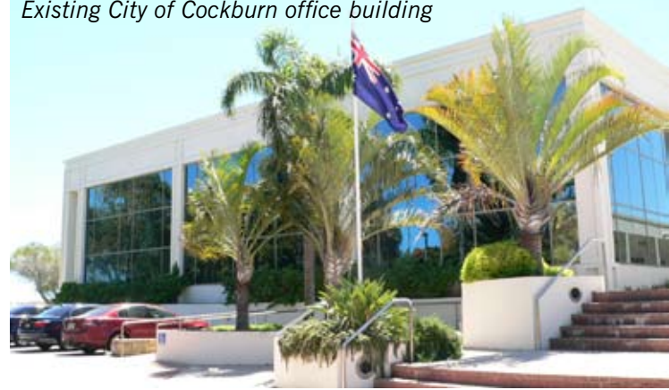
Existing City of Cockburn office building
