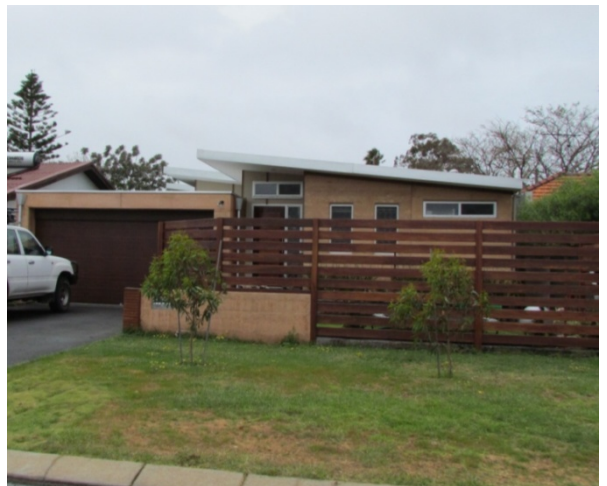
Skillion Roof Late 50/60's
