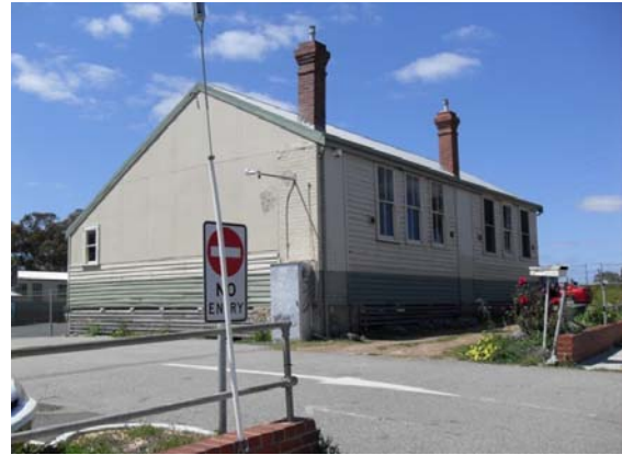
Figure 17 Original Hamilton Hill Primary School Building Source: City of Cockburn Local Government Inventory
