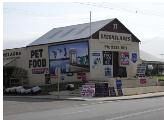
Figure 20 Greenslades Building Source: City of Cockburn Local Government Inventory
