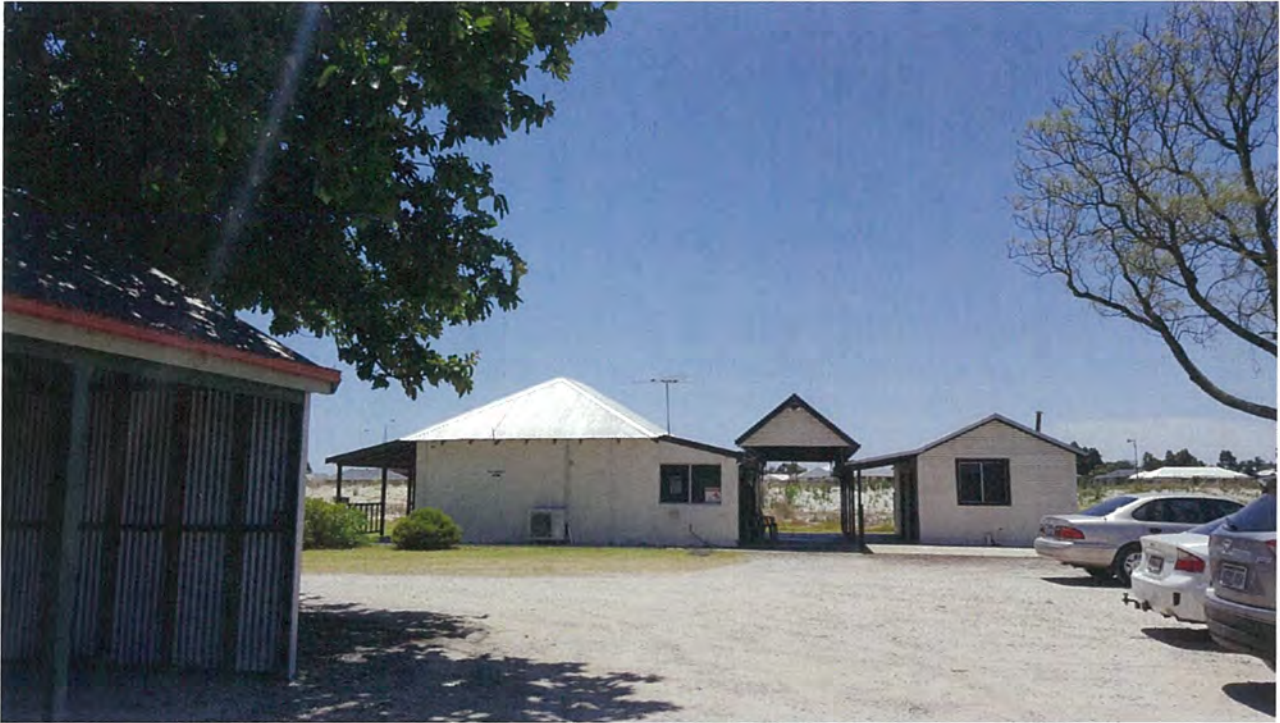
Figure 2. Photo of former dwelling and connected outbuilding, southern elevation
