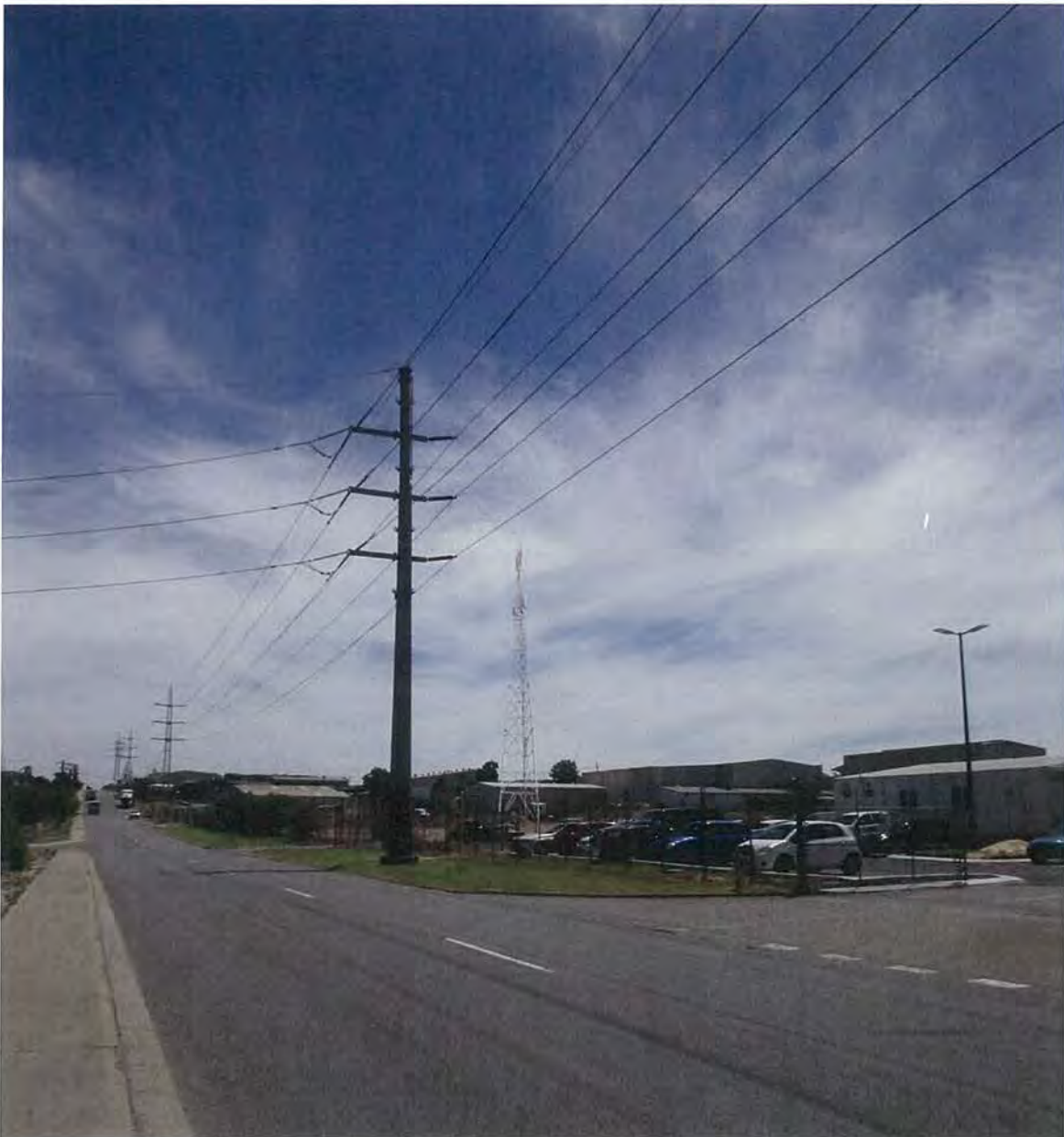
Looking north along Wellard Street (source Aurecon)
