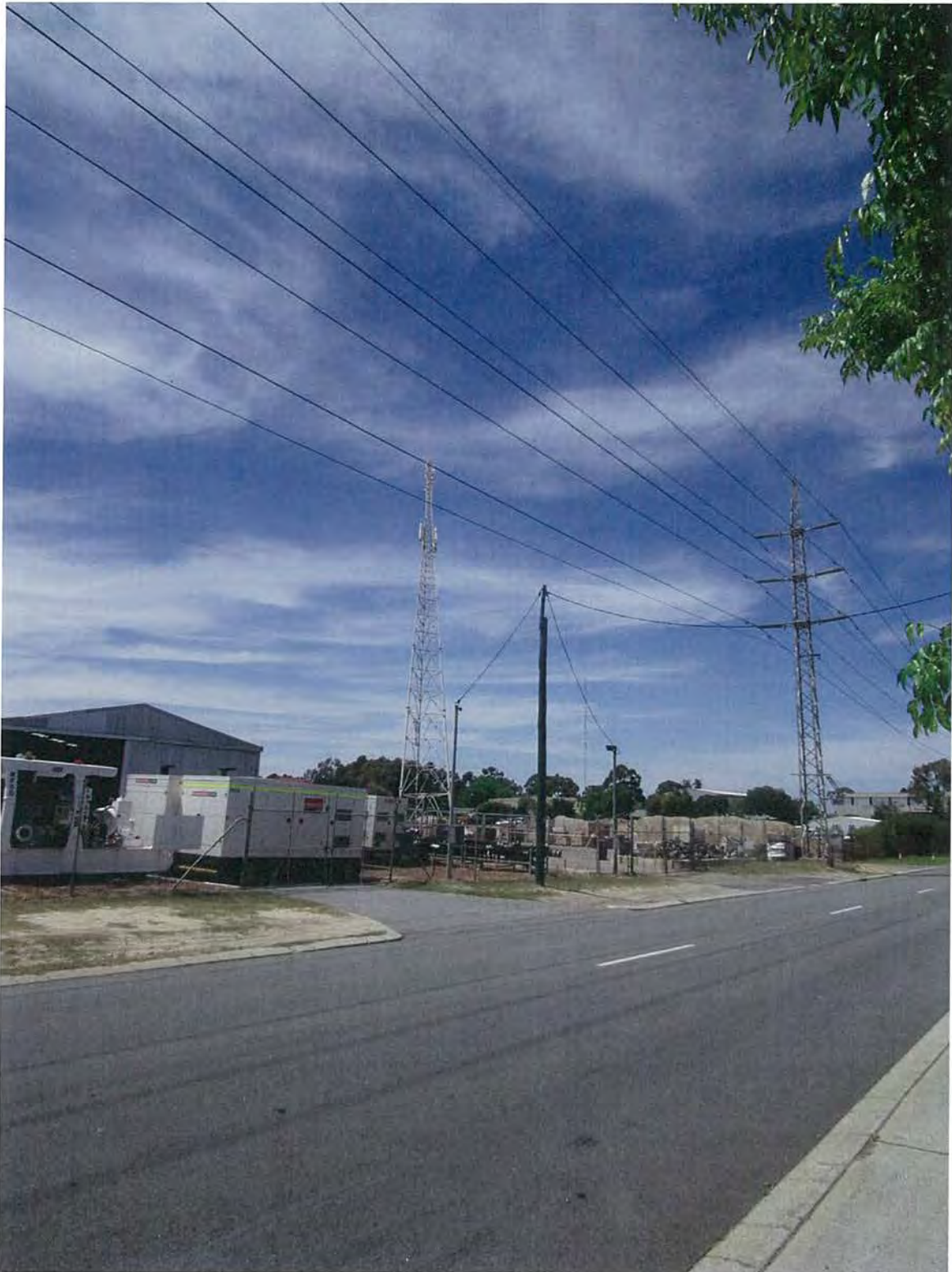
Looking south along Wellard Street (source Aurecon)
