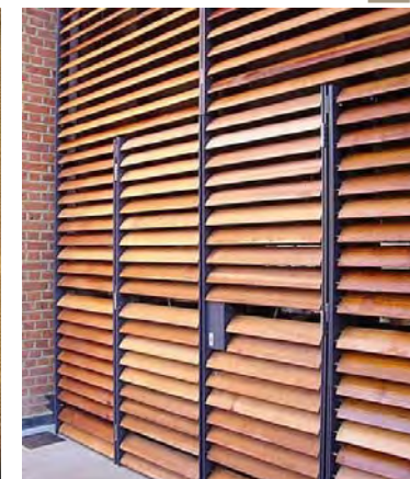
PLANT LOUVRE SCREENING AND VENTILATION.
