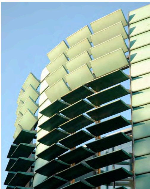
HORIZONTAL LOUVERS OFFER PROTECTION TO WINDOWS
