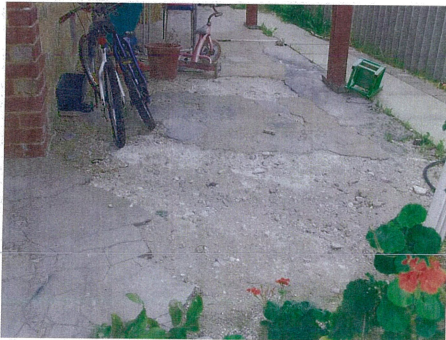
12. Deteriorated floor to the east verandah.
