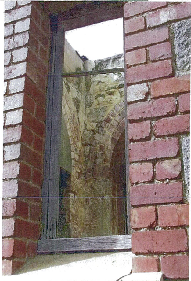
10. West window of the tower – view showing deteriorated brickwork and joinery, and interior deterioration.
