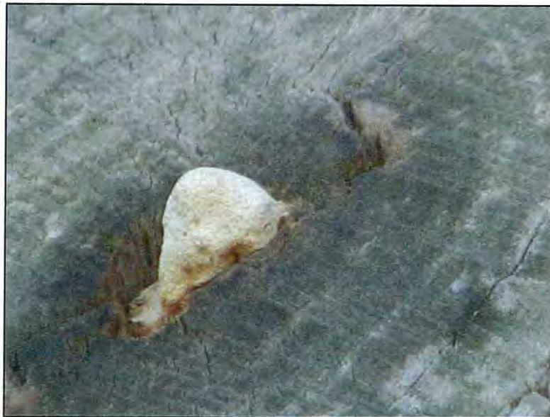
Image 5 – Early development of decay fungi sporophore (fruiting body).
