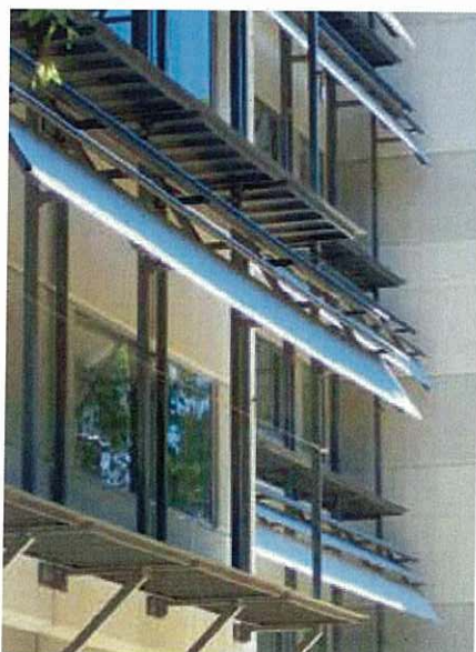
Adjustable shading devices can seasonally adapt
