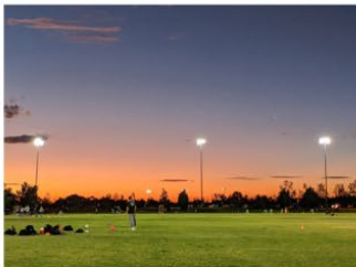
SPORTING FIELD WITH FLOOD LIGHTS
