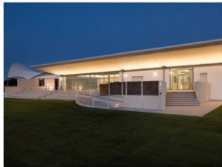
ACCESS TO OVAL FROM CLUB ROOMS
