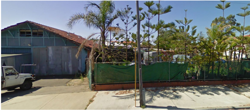
Plate 27. 2009 - South boundary of the Project Area (Courtesy of Google Maps)
