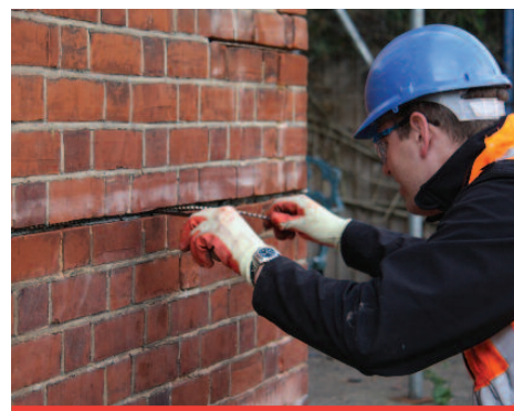
HeliBar is inserted into HeliBond grout within a cut slot
