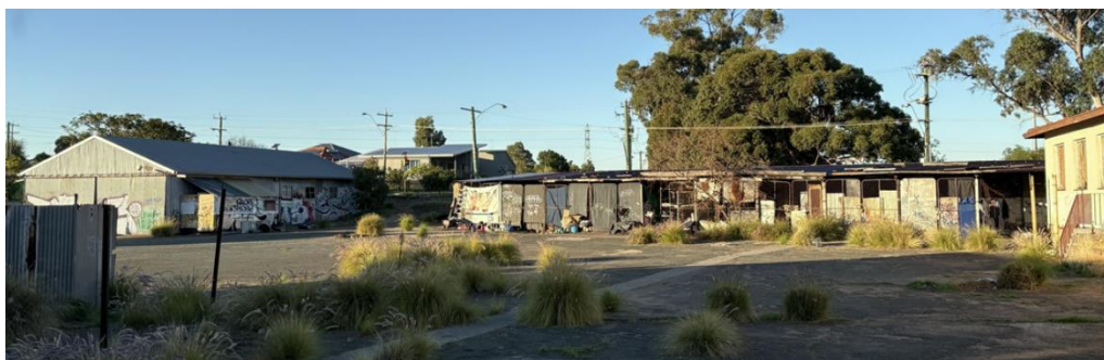
Structures 3 and 4 – to be demolished
