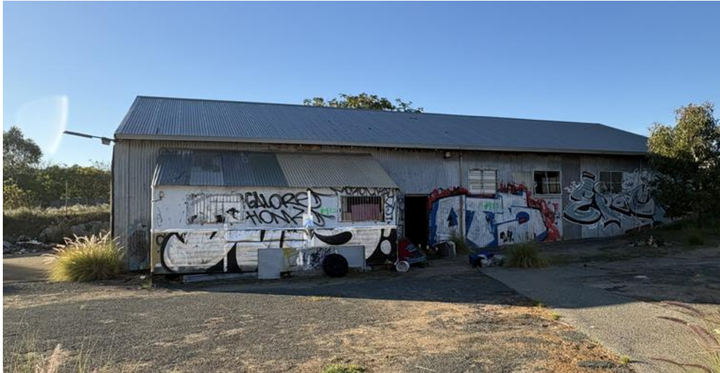
Structure 3 – to be demolished
