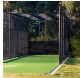
Six cricket nets (2 relocated from across site, 4 new), with storage shed, with an adjacent storage shed
