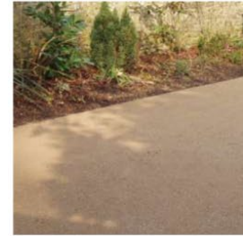
Stabilised compacted gravel path surface, to areas where site or tree locations are more restrictive
