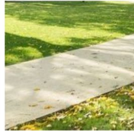
Broome finished concrete paving perimeter circuit path - connecting onto existing footpaths
