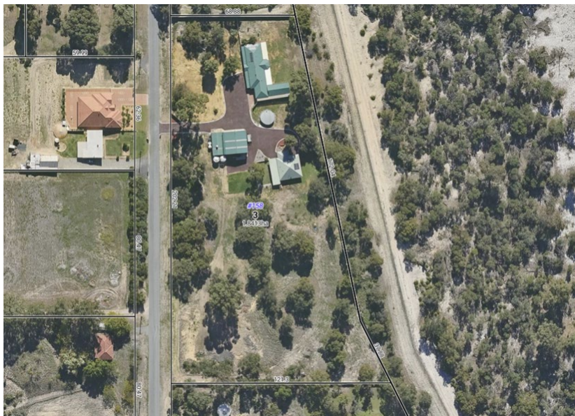
Image 4 – Site Context – Aerial
