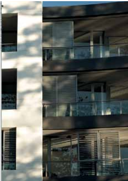
A combination of open, solid and adjustable elements facilitate optimised airflow
