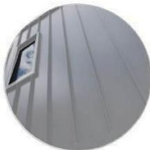
Profiled Metal Cladding (Colorbond WALLABY)
