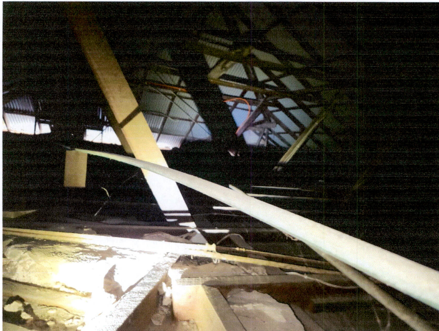
Figure 3 Roof struts supporting the roof frame is sitting on the internal walls
