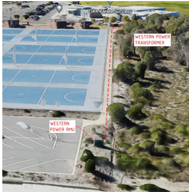
Image 3 - Indicative location of existing underground high voltage cable
