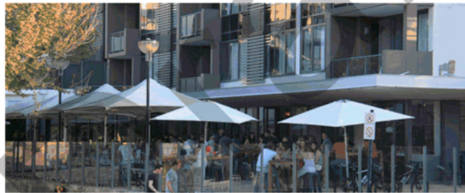
Mixed use development will encompass active street edges that create a comfortable pedestrian environment
