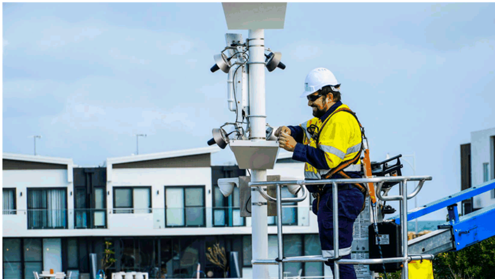
Image 5: LED streetlight upgrade, Port Coogee, June 2020
