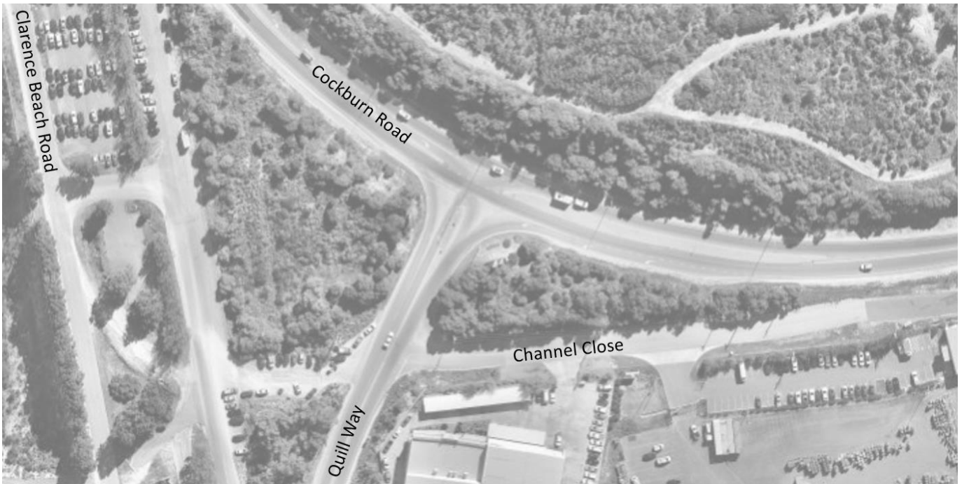
Figure 27 Intersection of Cockburn Road and Quill Way (source: Nearmap)
