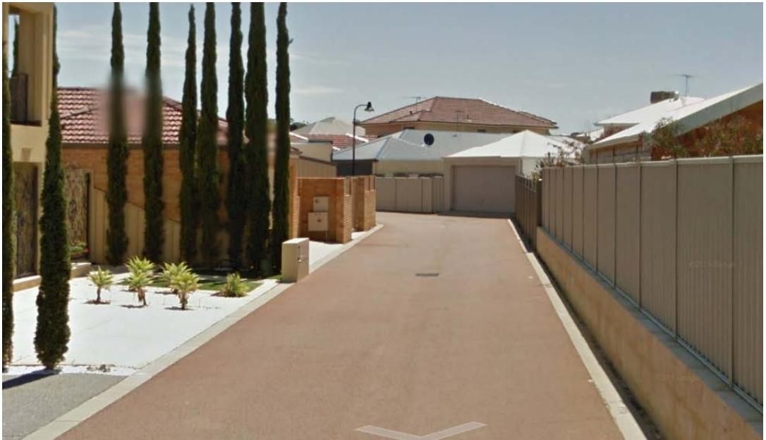
Figure 1 The bend in the laneway does not allow refuse truck drivers to see obstructions within the laneway before entering
